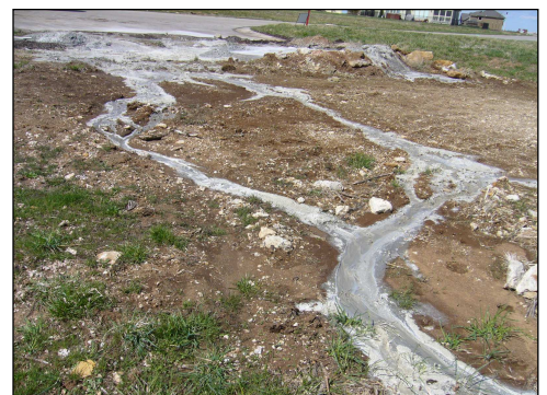
Unacceptable: Pit full and overflowing.
