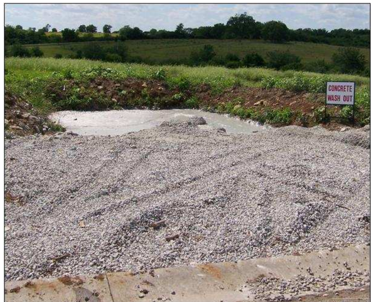
Excavated washout facility with signage and stabilized access.
