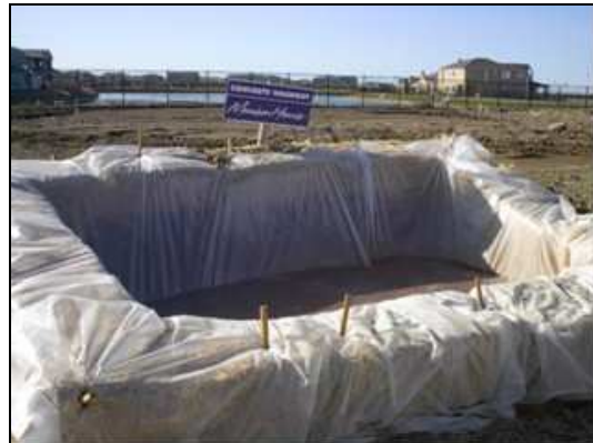
Self-installed washout container w/ 10-mil min. plastic.
