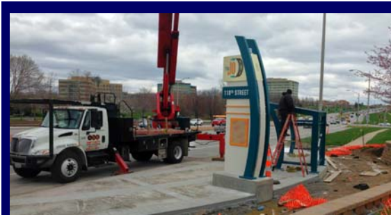
Bus Shelter under construction near 119th & Metcalf
