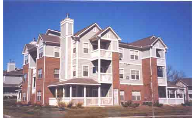
Figure 16— For all multi-family buildings and single-family attached townhomes, an amount equal to 40% of the total net exterior wall area of each building elevation, excluding gables, windows, doors, and related trim, shall be brick or stone.
