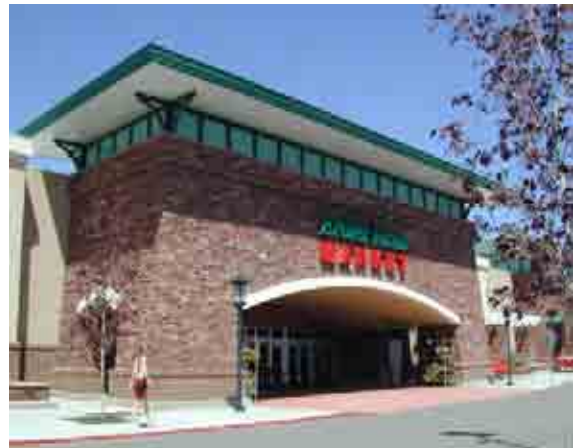
Figure 29— All primary buildings should be constructed or clad with materials that are durable, economically-maintained, and of a quality that will retain their appearance over time.
